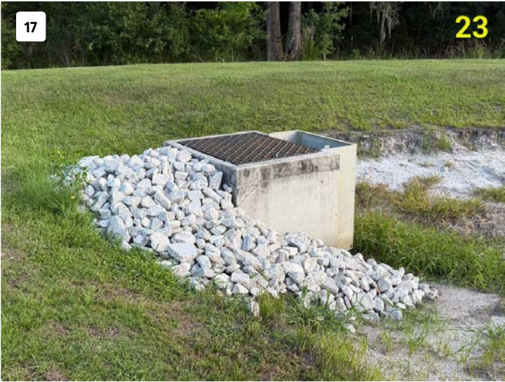
Pond 23 water control structure rip-rap Installation of 2 tons of rip rap to armor the structure from erosion.
