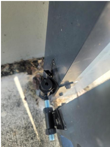
Lower hinge — detail
