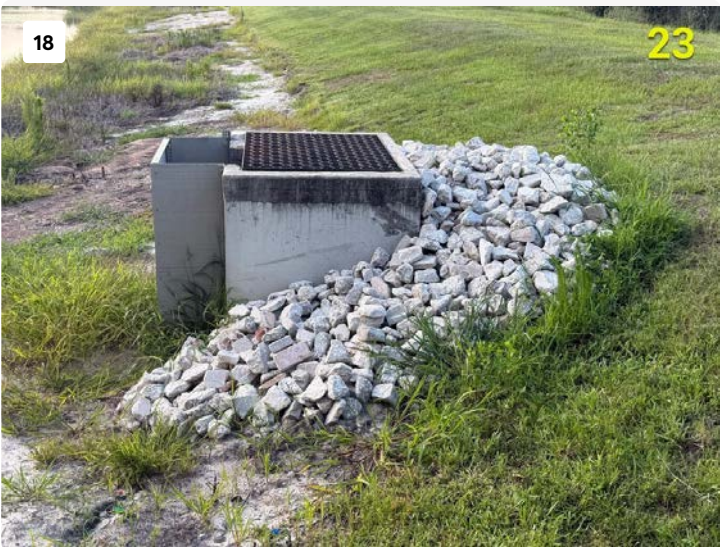
Pond 23 water control structure rip-rap Installation of 2 tons of rip rap to armor the structure from erosion.
