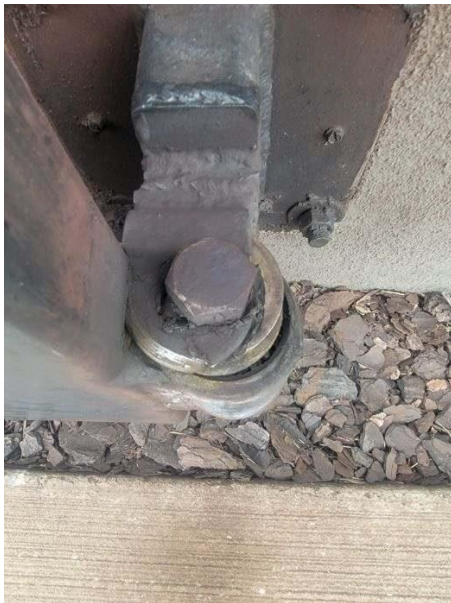
Bottom hinge — detail
