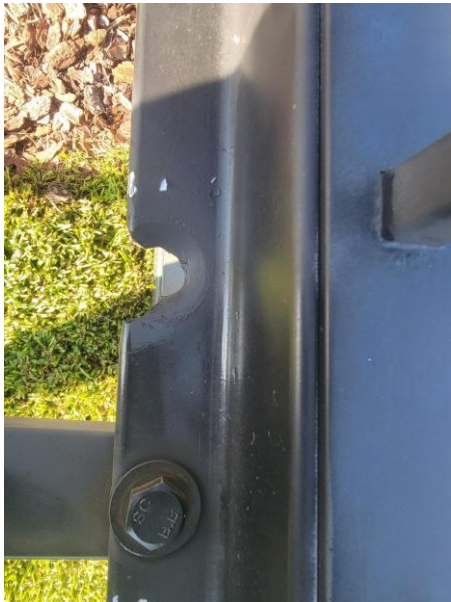
Re-drilled operator mounting holes
