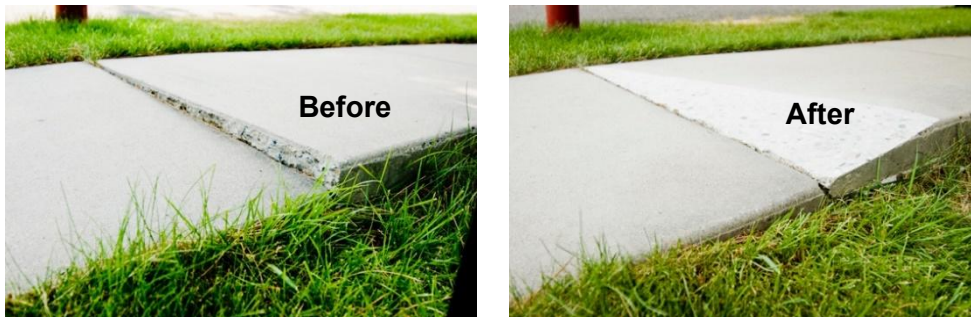
Figure 9: Precision Sidewalk Safety Work Example
