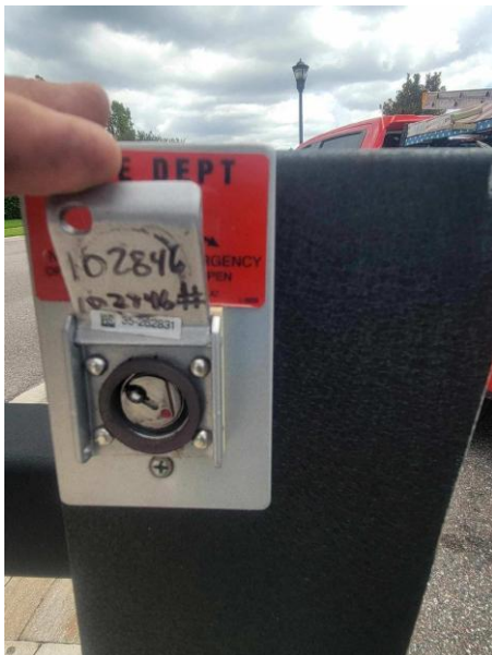
Fire key number recorded during inspection
