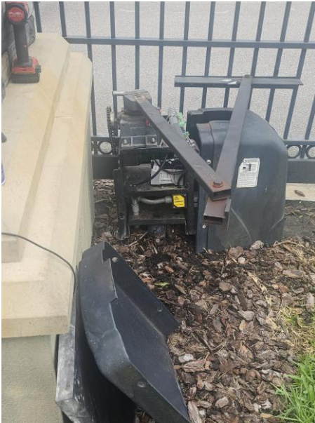
Bent operator mount
